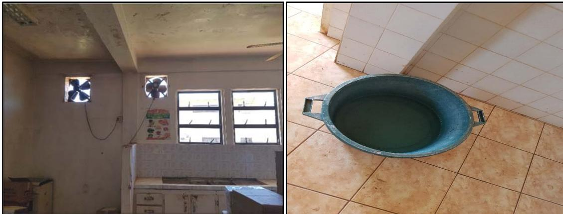
Figs. 6 & 7 - Leaks from the ceiling at Lethem Hospital Laboratory
