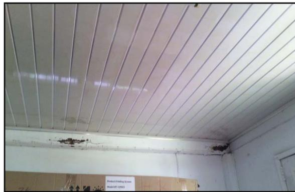
Fig. 20 - Termites on the ceiling at Mahdia Hospital Bond
