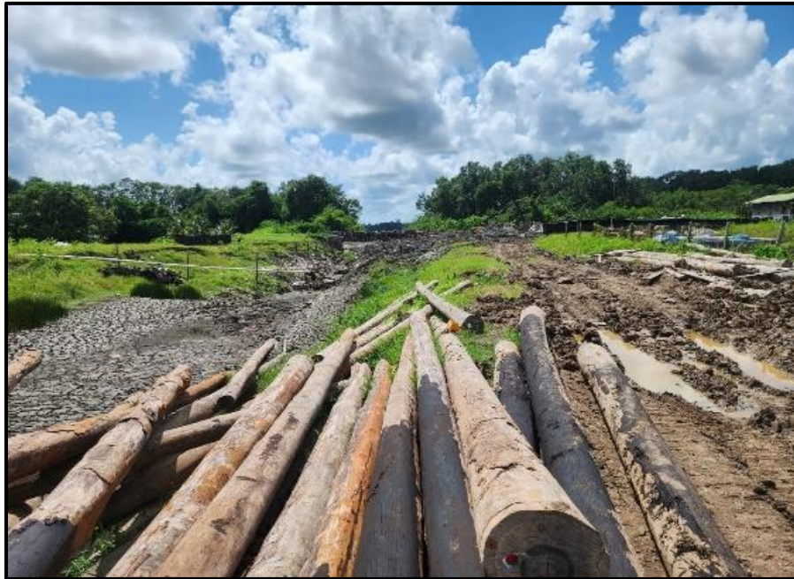
Photographs of the inactive site at Belle Vue Pump Station - 14 August 2024
