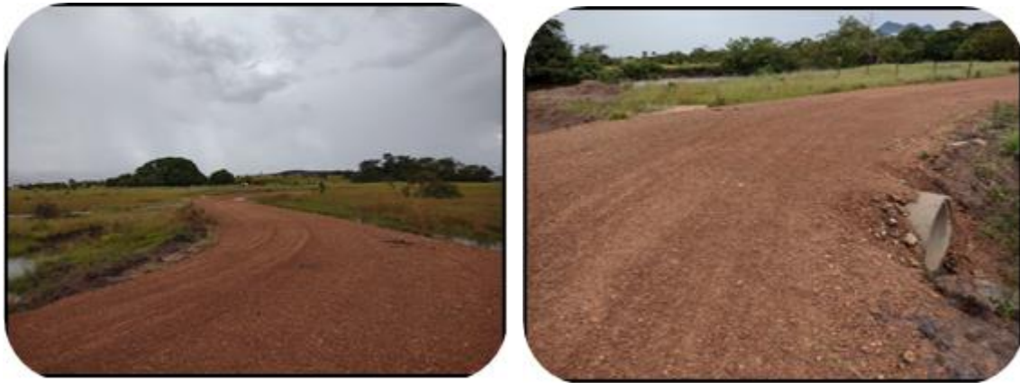
Photographs of the completed roadworks at Shiriri Village - 13 July 2022
