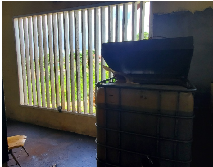
Image showing fuel container placed next to vented wall
