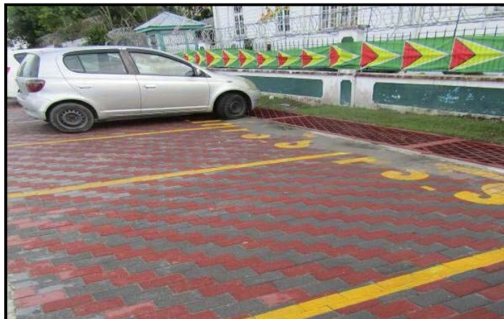
Newly Constructed parking lot
