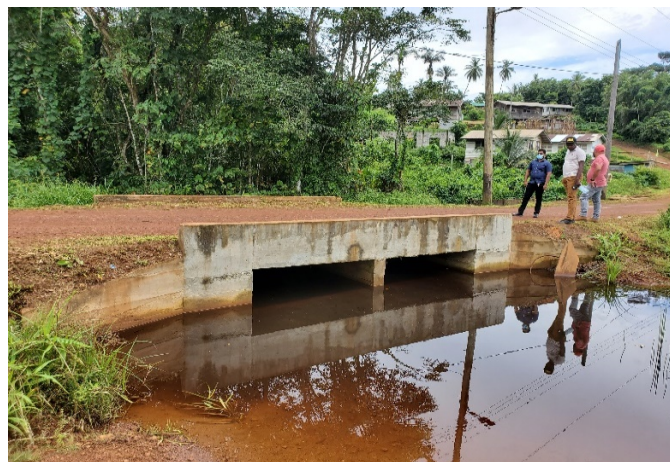
Image showing the completed Thomas Hill bridge
