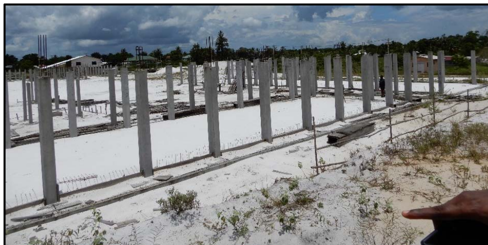
Construction of Yarrowkabra Secondary School
