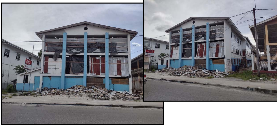
Ongoing works at Smyth Street
