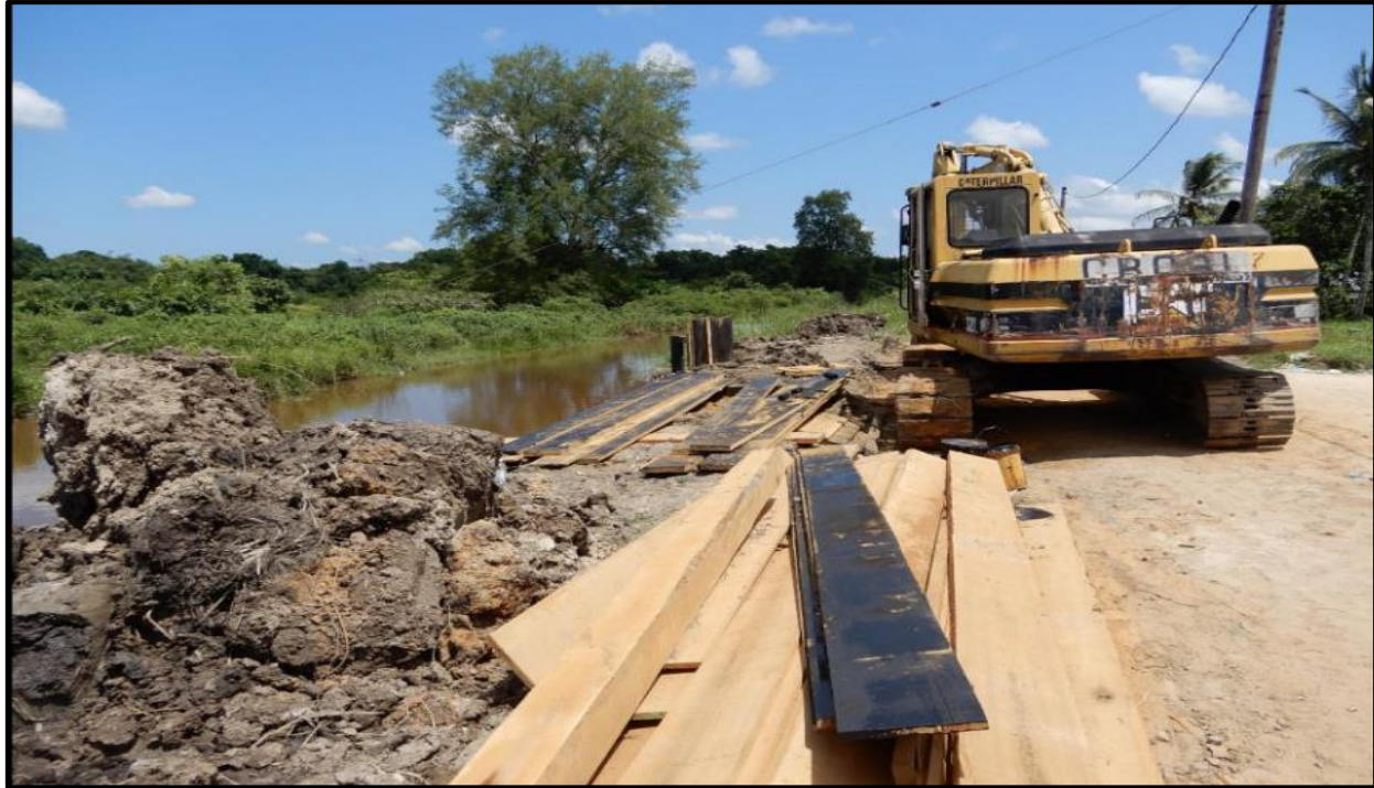
Work in progress on site - 8 October 2020
