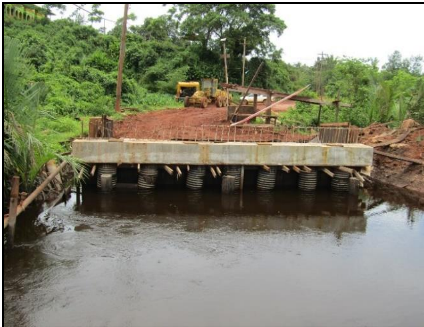
Only two reinforced concrete abutment for the bridge completed - 15 August 2019
