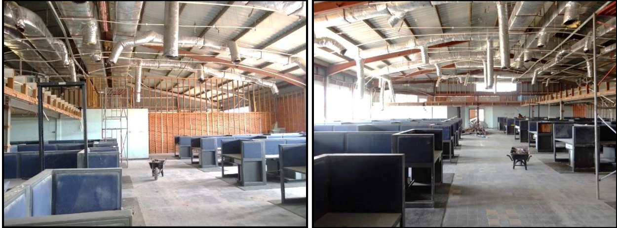
Demolition works in progress to the interior of the building - 4 September 2020
