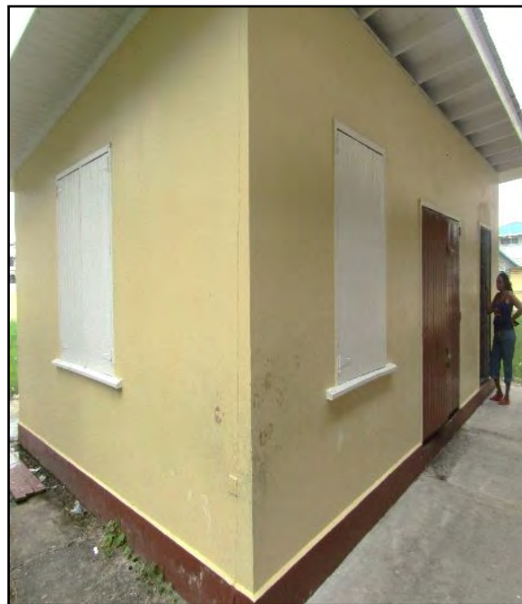
The wooden windows installed
