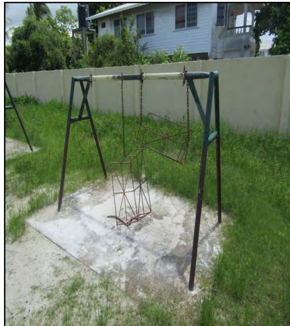
Poorly constructed swing- cost: $415,000
