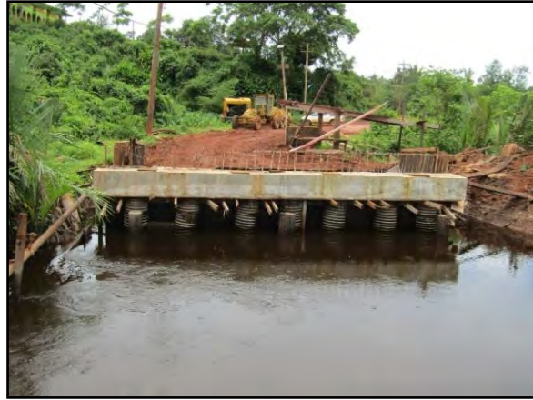
Only two reinforced concrete abutment for the bridge completed
