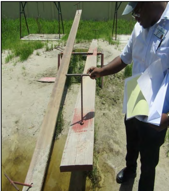
Poorly constructed inferior sea saw- cost: $205,000
