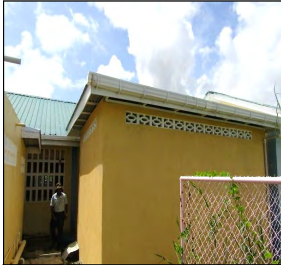
Newly constructed stores building completed using recurrent budgetary allocations
