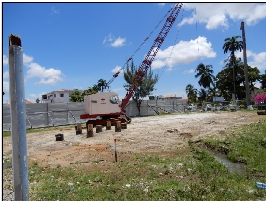
Piles for foundation and one piece of equipment
