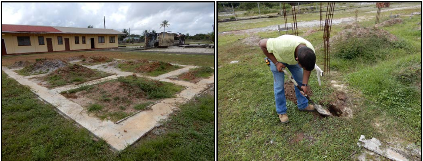
The abandoned site with two separate foundation works
