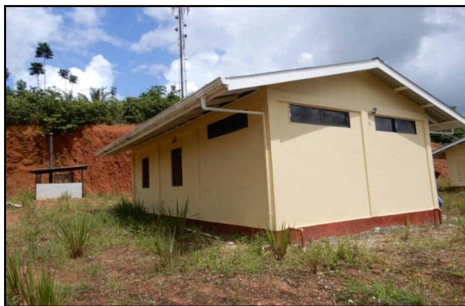
Incomplete Mortuary Building
