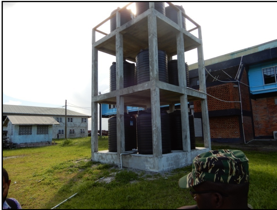
The completed trestle
