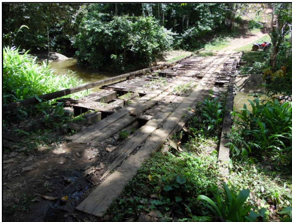
The old existing bridge still on site
