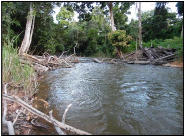
The old collapsed bridge - Kawa Creek
