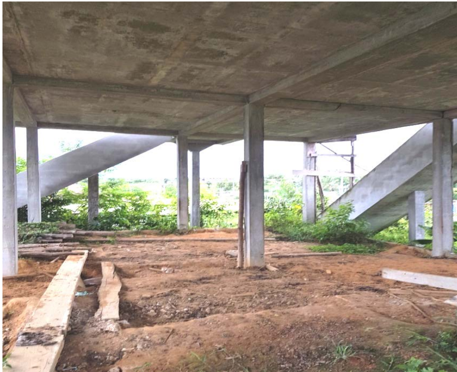
Construction of one Duplex Living Quarters on Mongrippa Hill, Bartica
