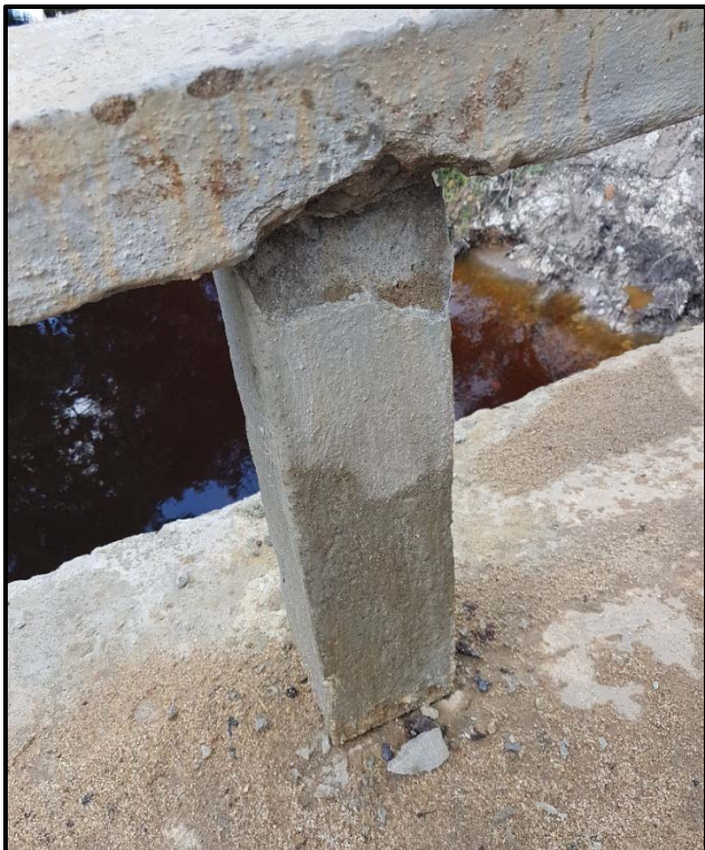
Shoddy works to reinforced concrete bridge rails
