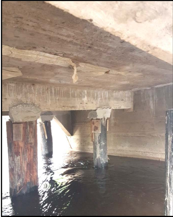
Additional piles installed to bridge at a total cost of $2,998,000 that are wedged to the underside of the beams and are bearing no loads from the bridge structure.
