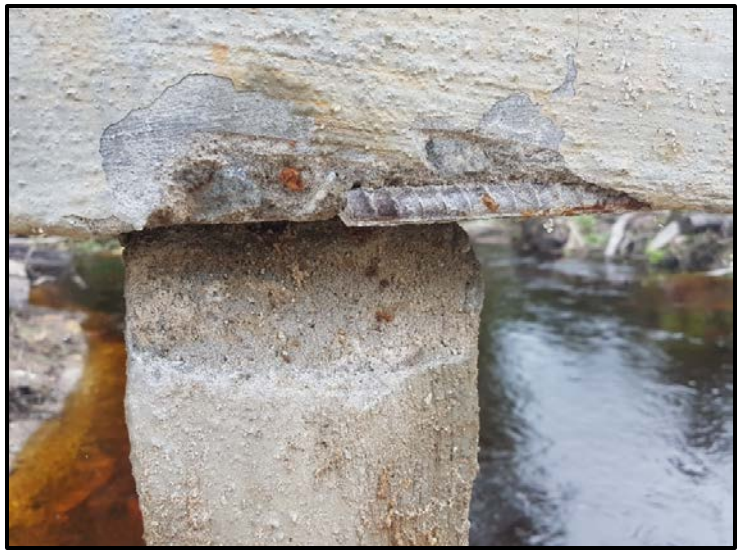
Shoddy works to reinforced concrete bridge rails
