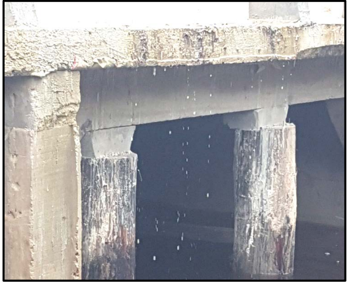
Additional piles installed to bridge at a total cost of $2,998,000 that are wedged to the underside of the beams and are bearing no loads from the bridge structure.
